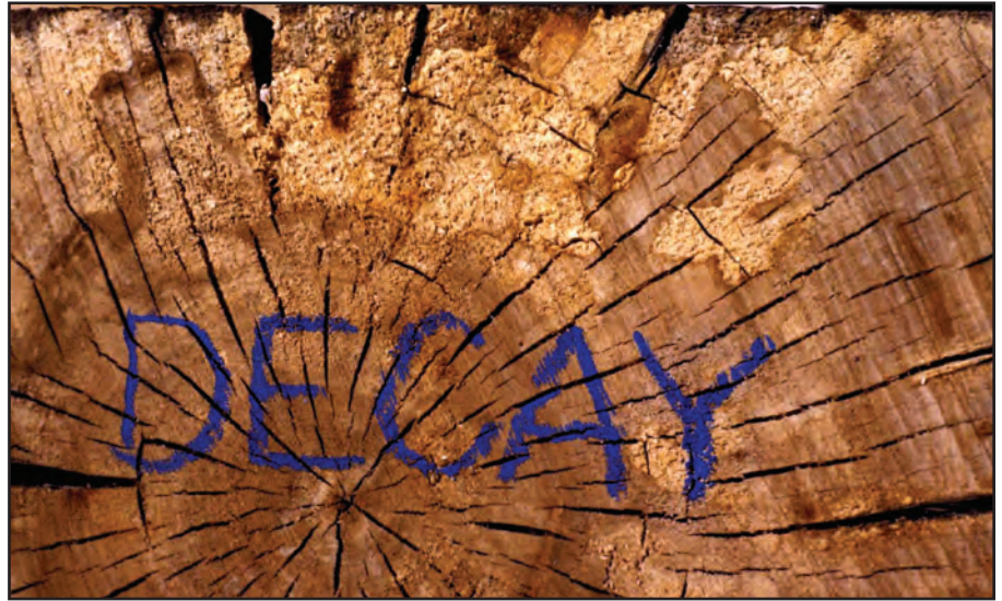
Figure 18. Decay in an air-dried crosstie.
