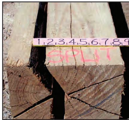
Figure 29. This tie has a split that is over one inch wide, and it's not salvageable.
