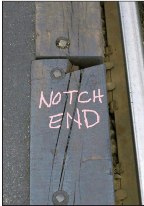
Figure 33. The miscut end should have caused this tie to be culled. This cut is from the felling notch in the woods.
