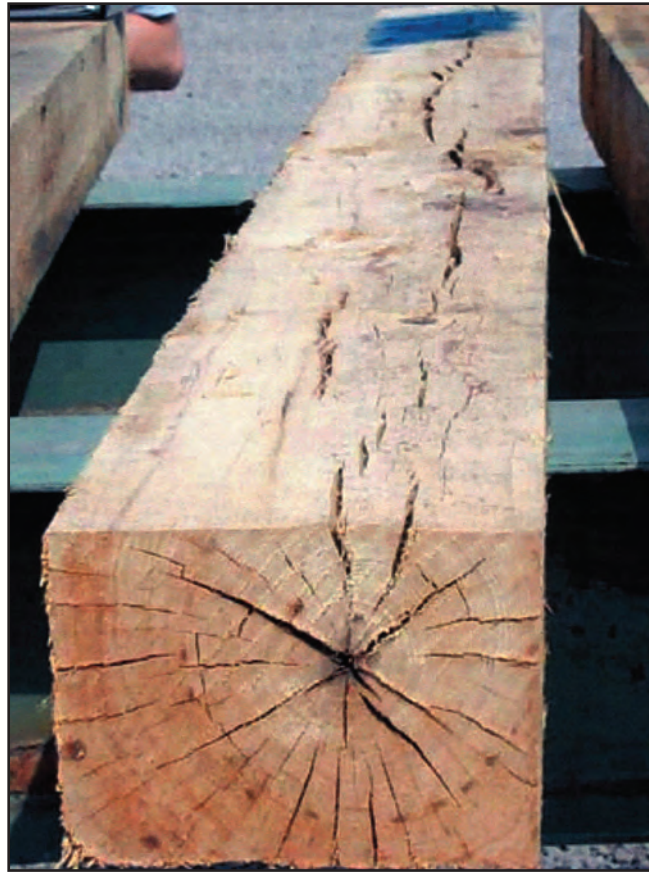
Figure 26. This tie would be rejected because the long check in the middle of the tie is over half the length of the tie, and it is 1\frac{3}{4} " deep.
