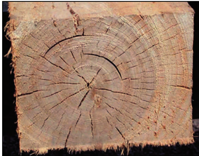
Figure 23. The combined width of these two ring shakes is 4", which causes rejection under a 9" face width.
