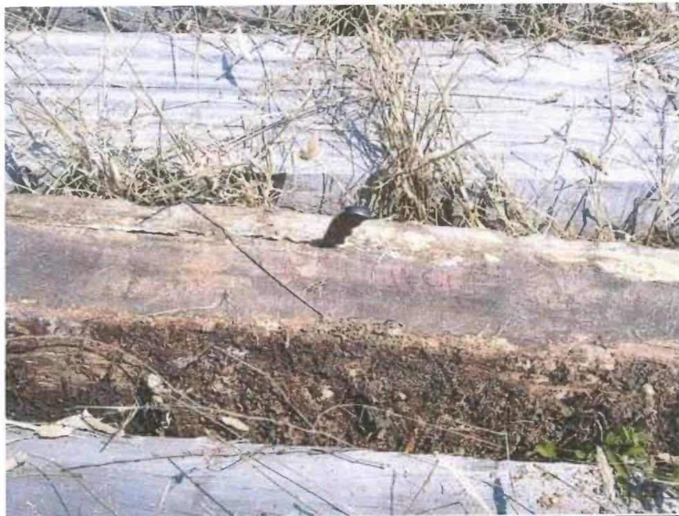
**Figure 5** - Tie #9 (Turada) with substantial decay which appears to be in a sapwood zone.
