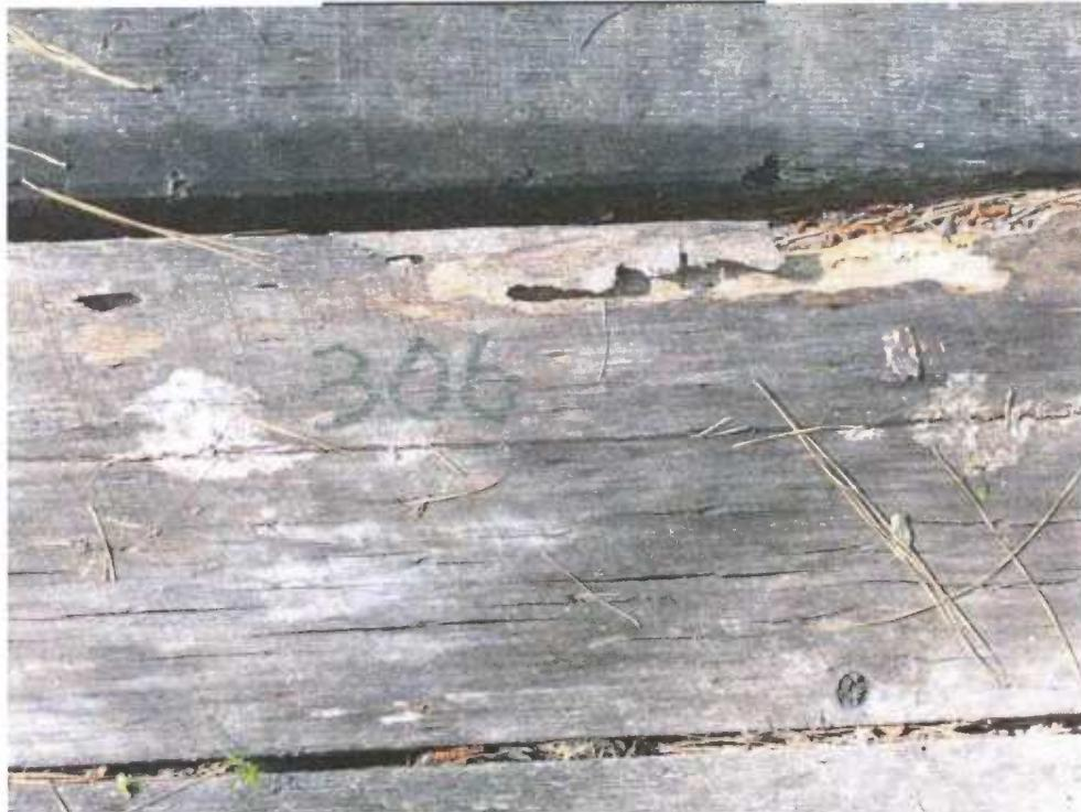
**Figure 3** - Tie #306 (control) showing severe decay and beetle damage.
