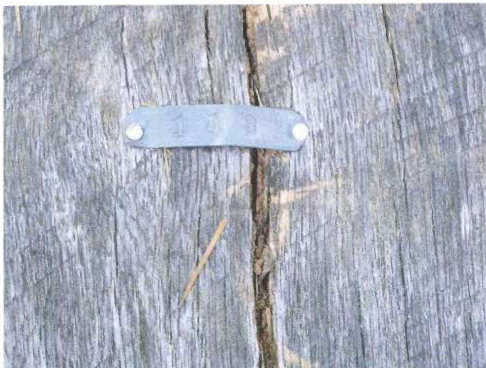
**Figure 4** - Tie #148 (red oak/control) with termite shelter tubes in check and surface grazing by termites.
