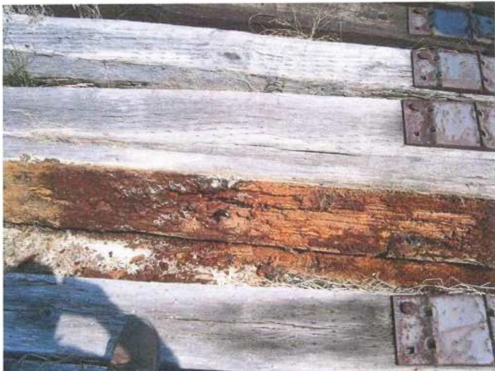
**Figure 7** – Tie #334 (untreated red oak) with extensive decay.
