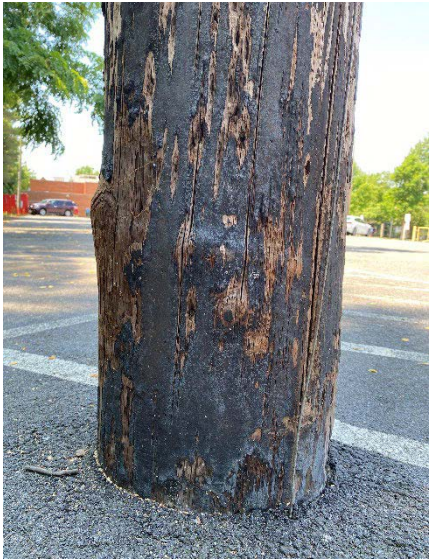
Figure 2.—Approximately 75-year-old creosote-treated pole in parking lot in Vienna, Virginia.
