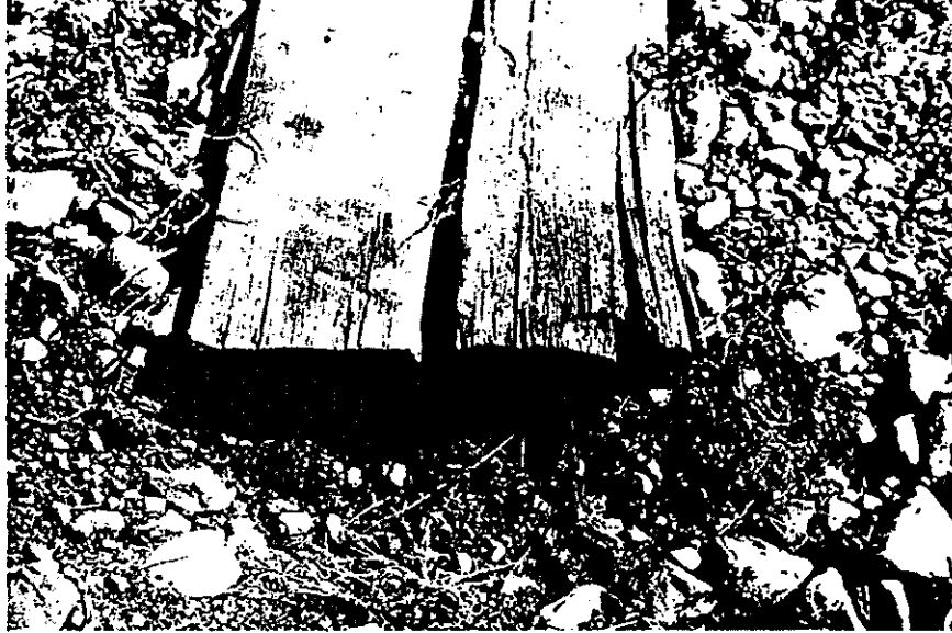
Figure 3. South End of Control Tie Number 7, Showing a Typical Split that was Only 1/16 Inch Wide at the Time of Installation in 1964.
