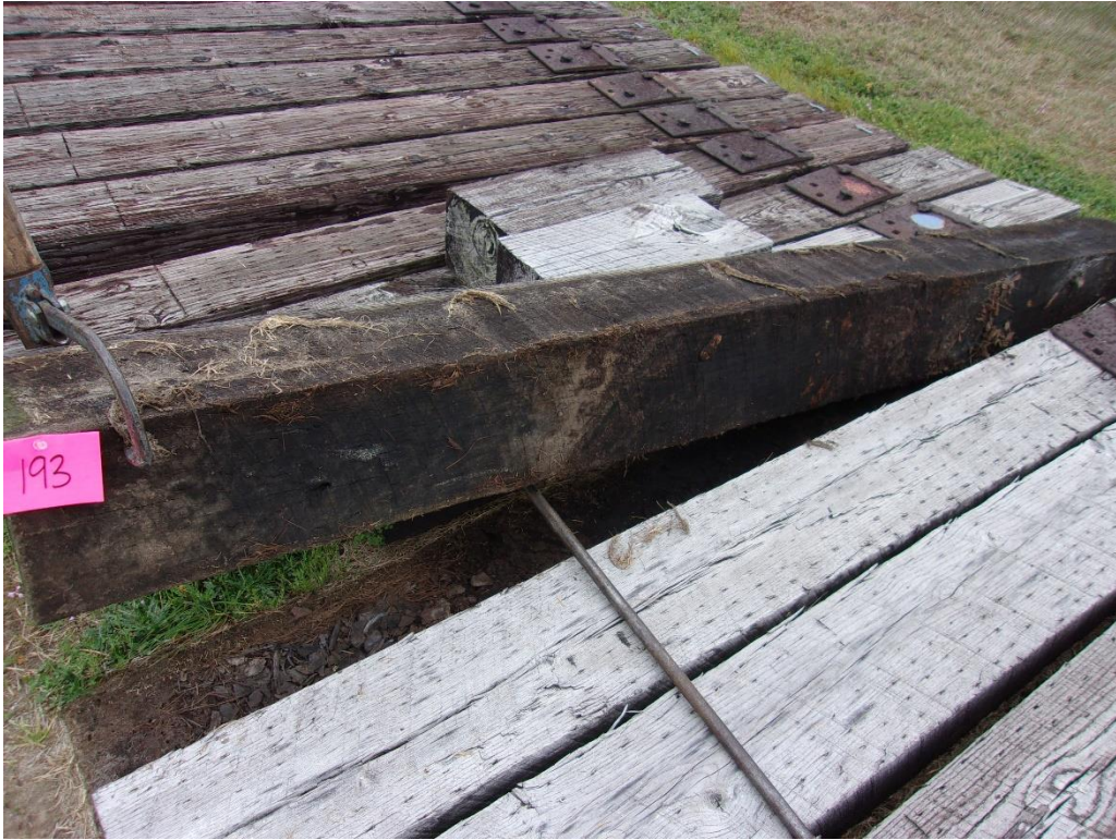
Figure 93 – Tie #193 white oak/borate/creosote/6lbs (Koppers).
