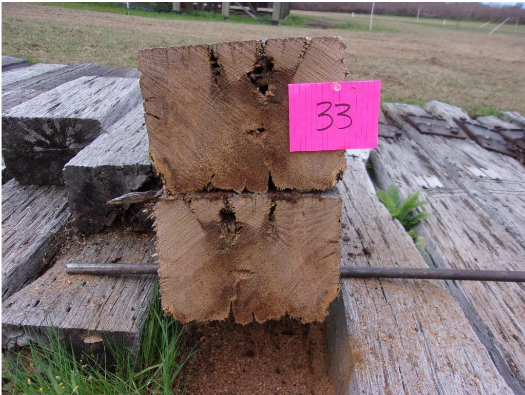
Figure 60 - Tie #33 untreated white oak with decay visible in cross-section.
