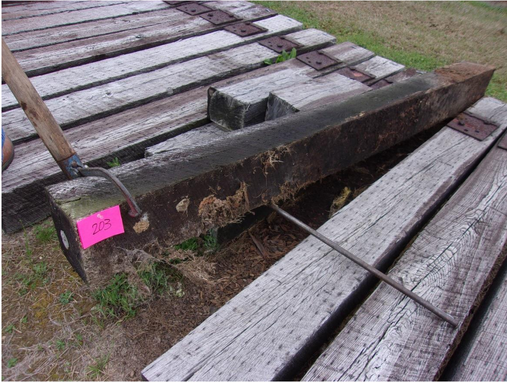
Figure 95 – Tie #203 white oak/borate/creosote 7lbs (Koppers).
