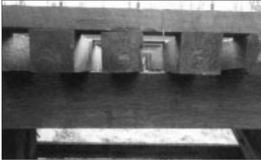
The use of Parallam® ties by the B&P Railroad represents the first application of the material in a railroad environment.
