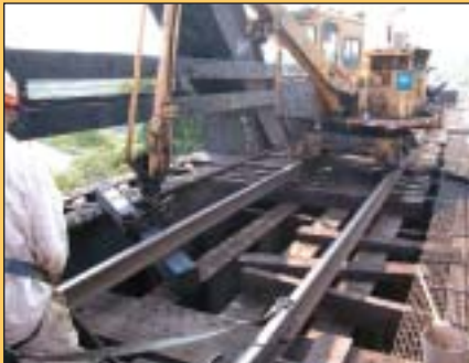
Replacing ties at this height is slow, methodical work. The strap attached to rail and the personnel is known as a rail slide and anchors bridge personnel to the rail so that if a fall occurs they'll be saved from a long drop with a difficult ending.
