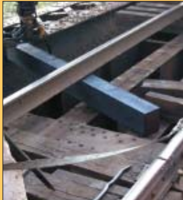
Replacing ties at this height is slow, methodical work. The strap attached to rail and the personnel is known as a rail slide and anchors bridge personnel to the rail so that if a fall occurs they'll be saved from a long drop with a difficult ending.
