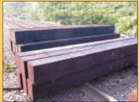
8"x10" bridge ties were the subject of the maintenance work.
