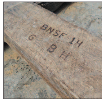
All ties are marked for the BNSF indicating the year and treatment type; this one will be dual treated with DOT (borate) and creosote.
